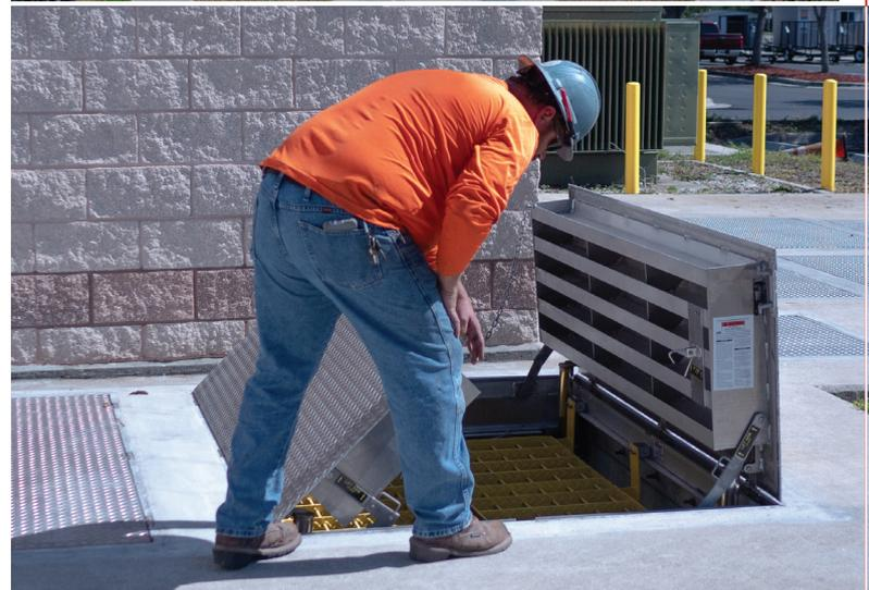
The new doors carry a 25-year warranty and are equipped with type 316 stainless steel hardware for superior corrosion resistance and BILCO's patented lift assistance for easy, one-hand operation. BILCO's doors are frequently specified in projects where there is a concern of water or other liquids entering the access opening.
