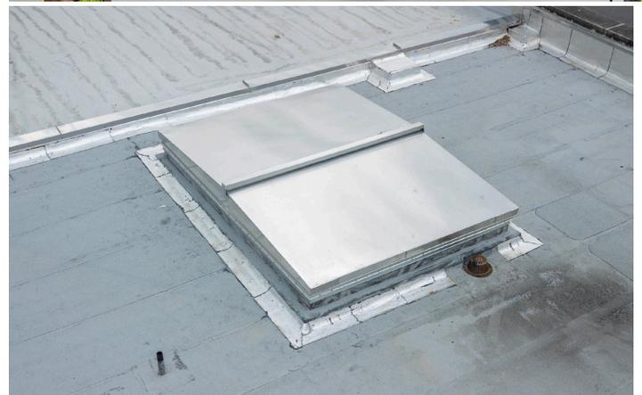
radiation source as necessary, without having to remove the equipment. "They will have to replenish the radiation source by going in through the roof, so this hatch allows them access to do that," Kersten said. "There isn't any other way to do that."
