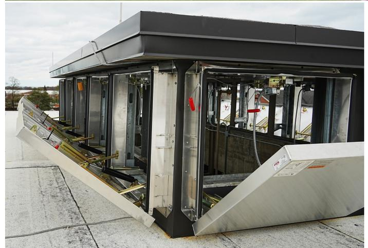
Smoke vents play an important role in helping firefighters bring a blaze under control. They protect property and aid firefighters in bringing a fire under control by removing smoke, heat, and gases from a burning building.
